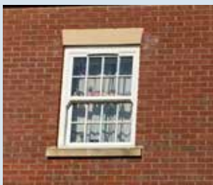
Sash window and lintel details
