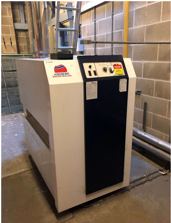
Picture - One of the existing Andrews Water Heaters
