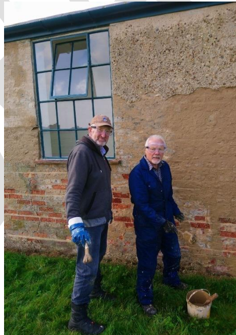
Volunteers applying a lime 'slurry' coat to Building 30 at Stow Maries Aerodrome, October 2021
