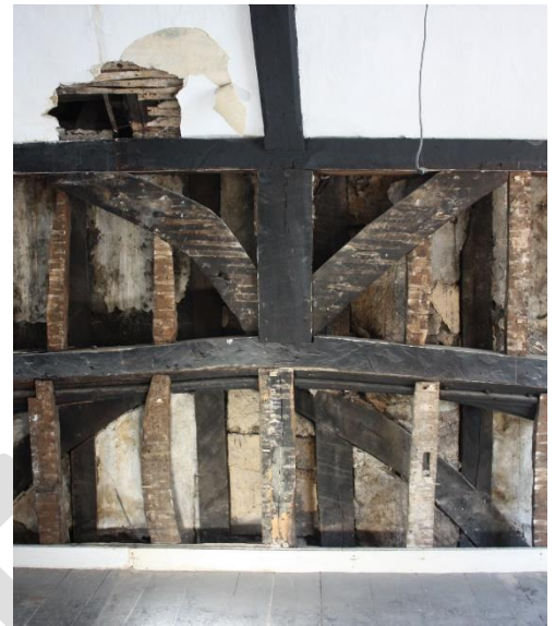
Photograph of medieval timber framing and wattle and daub taken 6 th of November 2020
