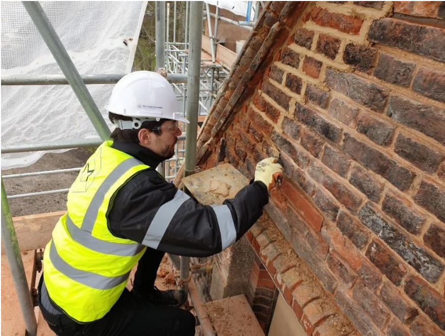
Cristian Petrescu of The Morton Partnership doing some lime pointing at Creeksea Place, Burnham-on Crouch in 2021
