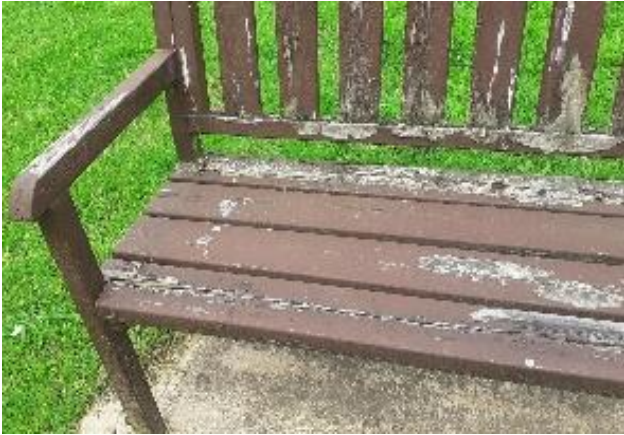
2a. general weathering of bench. This includes peeling paint and exposed timber.
