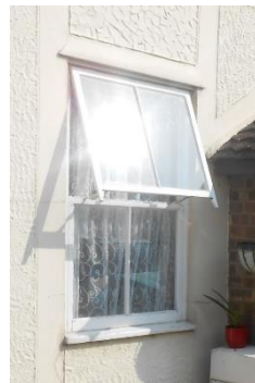
Fig. 27 – c.2003 timber tilt-opening sash-style window at No. 144
