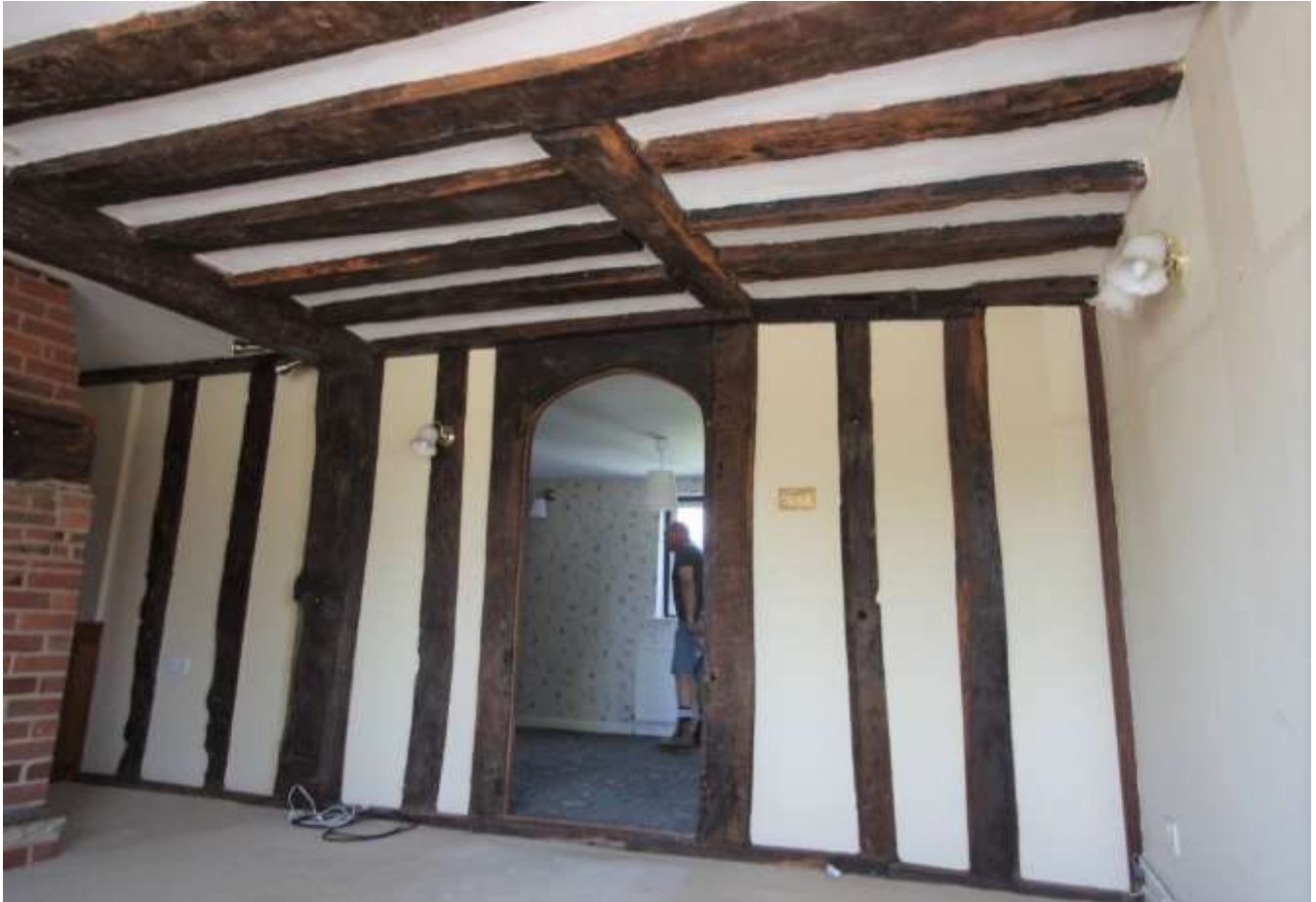
Photograph of the interior of Easthall Farmhouse, taken 16 th July 2015, showing original timber framing, a blocked stair trap, and a doorway with a four-centre-arched head.
