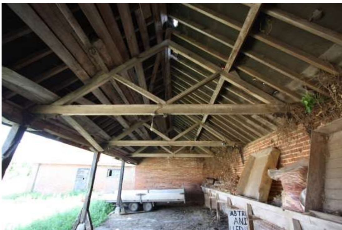
Internal view of the western byre at Easthall Farm, illustrating the pine roof structure, taken 16 th July 2015
