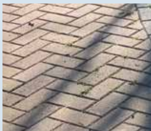
Herringbone brick paving
