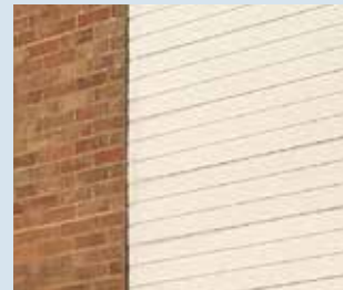
Mix of red brick and timber cladding
