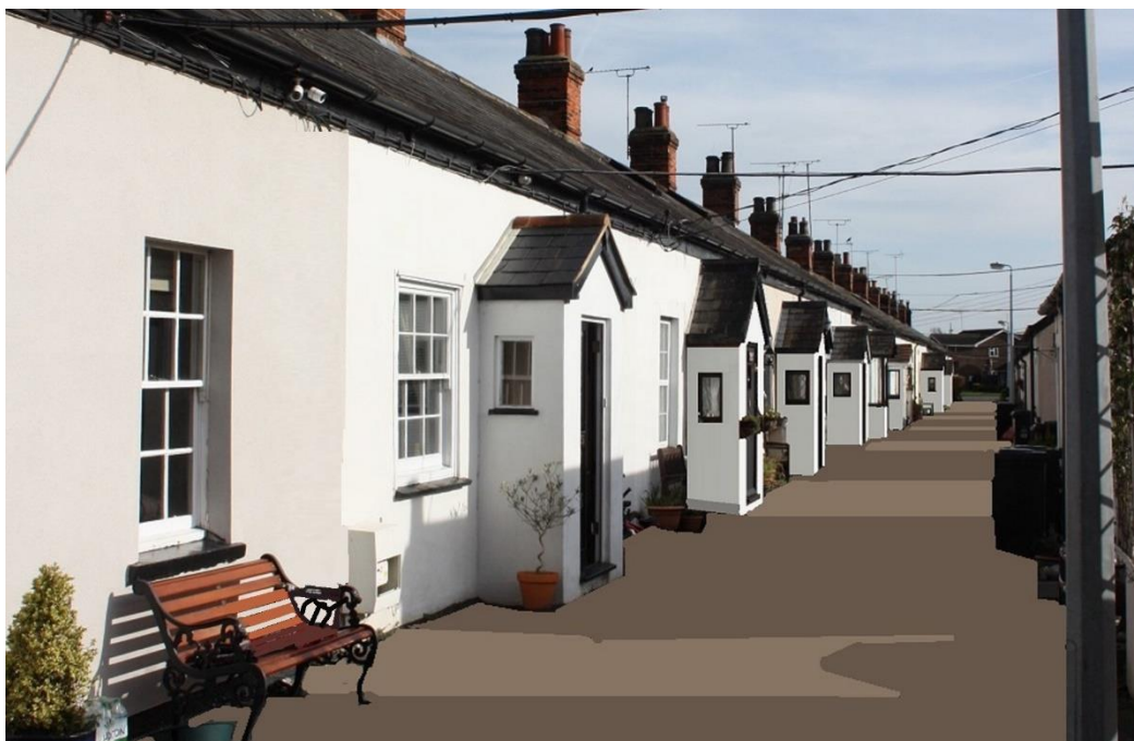
Fig. 45 – A mock-up showing the north row with render applied to the brick porches and a resin-bonded-shingle finish to the lane
