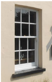
Fig. 22 – Original sash window at No. 140
