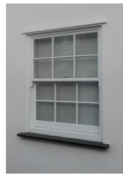
Fig. 29 – 2014 timber sash window with slim-profile double glazing at No. 155
