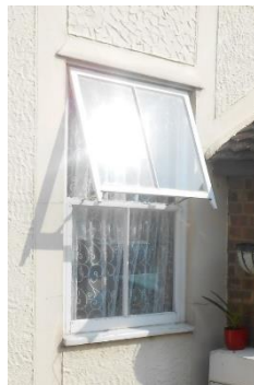
Fig. 27 – c.2003 timber tilt-opening sash-style window at No. 144
