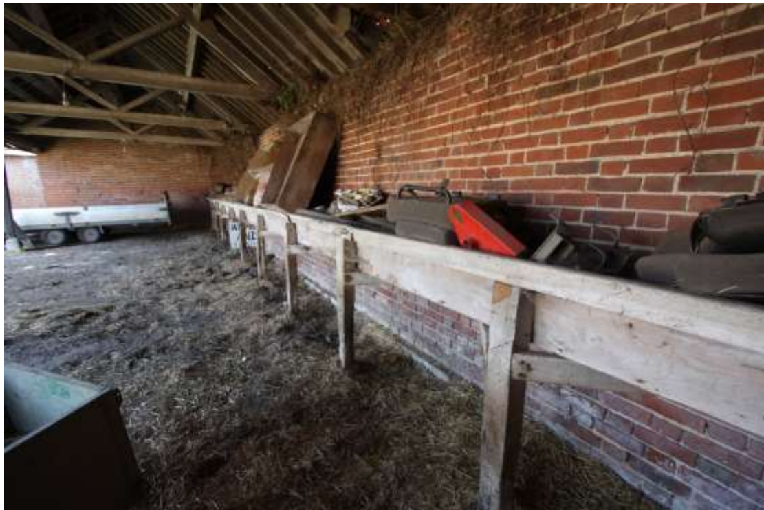
Internal view of the western byre at Easthall Farm, illustrating the original elm manger, taken 16 th July 2015
