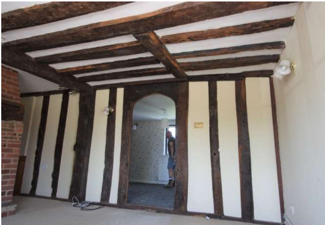
Photograph of the interior of Easthall Farmhouse, taken 16 th July 2015, showing original timber framing, a blocked stair trap, and a doorway with a four-centre-arched head.
